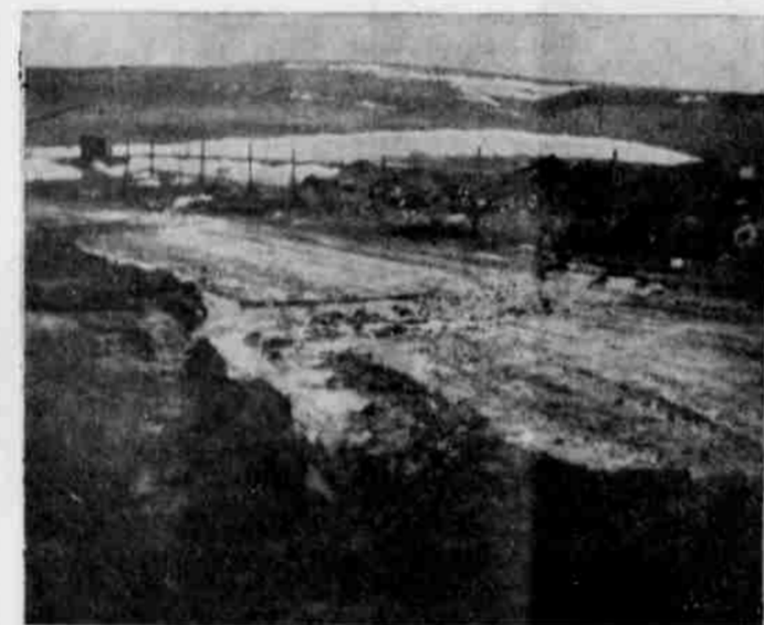
ROADS SUFFERING—This photo shows how the water running across the Balm Fork road near the Heppner dump has cut into and damaged road. Hundreds of other similar cases can be found on nearly every road in the county. In the foreground the stream has cut a ditch over three feet deep into which the water is pouring. (GT Photos)
