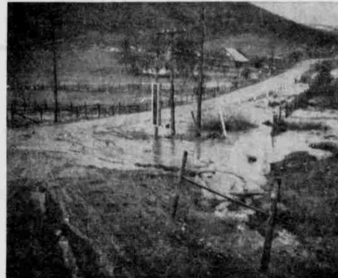
MUD COVERED HIGHWAY just south of Heppner on the Condon road. Topsoil washed from fields has completely filled ditches and overflowed several inches deep on the highway. This is one of the pictures taken a week ago during the very heavy runoff and similar scenes could be found on nearly any road in county.
