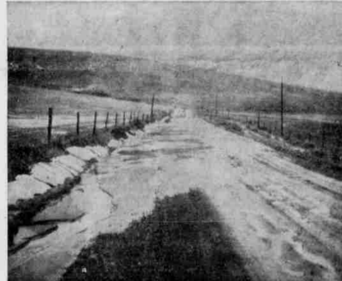
BALM FORK ROAD, shown covered with mud from adjacent fields for a stretch of over 100 yards was just one of the many instances of heavy runoff and soil loss that could be found throughout the county as a result of the snow melt and rains early this week. The mud in this photo was as much as 8 inches deep on the road and ditches were full.
