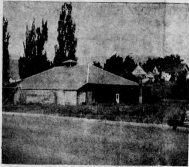
DOOMED—Heppner's old civic center building, the center of considerable controversy over the years, is one of the buildings which will eventually be torn down as a result of Wednesday's election which gave voter approval to a plan to remove all buildings on the north Main street property and make a public park out of the site. One end of the building has been remodeled in recent years and is being used to house the kindergarten classroom. (GT Photo)
