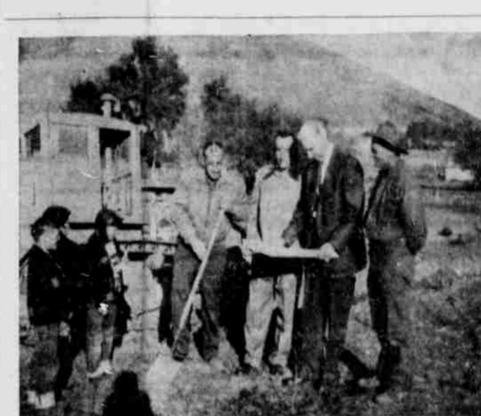
THE DIGGING STARTS —A great event took place Monday afternoon, when actual excavation got under way for the new Heppner grade school. The three young boys watching Ed Dick, school board chairman, turn over the first shovel full of dirt acted as though they didn't quite believe what they saw. They will be housed in the new building next year. Shown are left to right, Ed Dick, Edgar Collison, board member; H. C. Reed, superintendent, and Doc Sherer, county road foreman who is supervising the operation.
