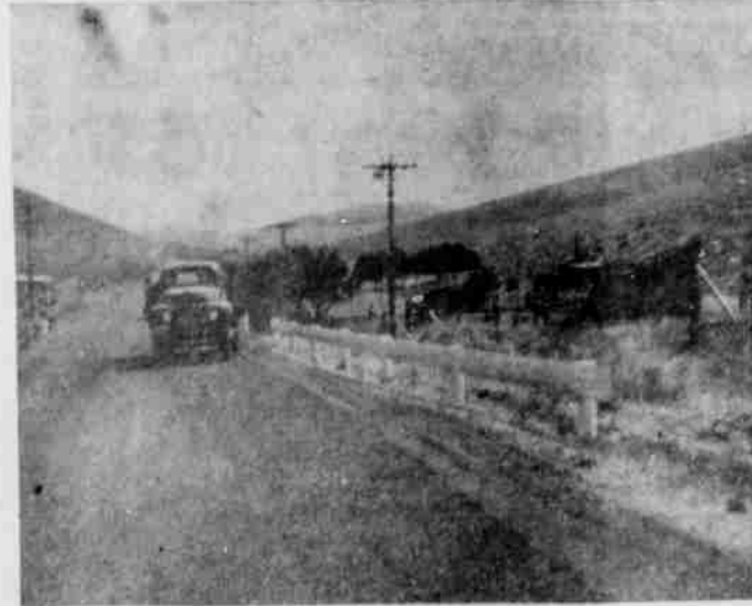
SOUTH HEPPNER BRIDGE where so many accidents have occurred is being given another safety treatment by the state highway commission. Since the last fatal accident there two weeks ago, the state has installed a new steel guard rail between the curve and the bridge, part of which shows in this photo, and has resurfaced much of that section of the highway to raise the outside of the road (add to the super) in an effort to help drivers stay on the highway and stop the many serious accidents at this point. The resurfacing was being done at the time this picture was taken, which accounts for the truck being parked on the wrong side of the highway. (GT Photo)
