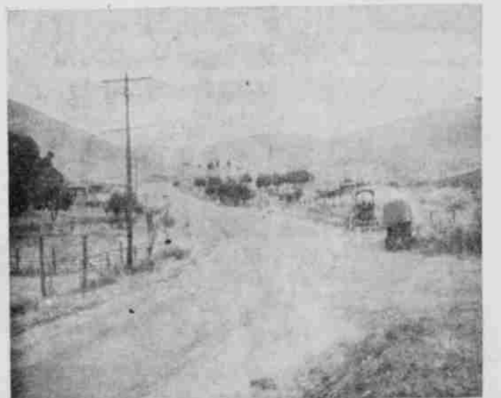
DEATH TRAP corner is shown in this photo of the highway turn on which there have been 18 fatal or serious accidents in seven years. Photographer was looking south, the direction of travel of all the cars involved in accidents. The bridge abutment is located about 150 feet past the end of the turn.
