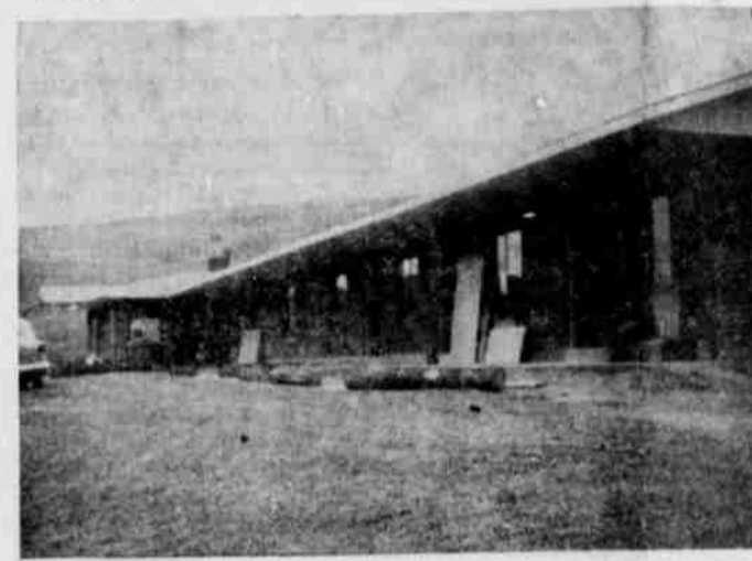
SIX MODERN UNITS—closeup of the motel reveals six one-and-two-bedroom units in addition to living quarters and office at the far end. Some finishing work and landscaping remain to be done, but when opened to the public, it will be Heppner's first motel. (GT Photo)
