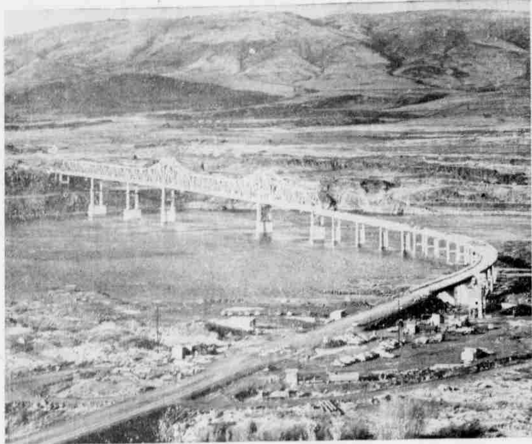
NEW INTERSTATE BRIDGE —The first interstate bridge across the Columbia east of Portland capable of carrying all loads will be open to the public December 18. Governors Paul L. Patterson of Oregon and Arthur B. Langlie of Washington will participate in joint ceremonies dedicating the bridge and celebrating first pour of concrete at The Dalles Dam. The Dalles interstate bridge, located about two miles east of The Dalles, is a direct link between Washington's Evergreen highway and Oregon's The Dalles-California highway and the water grade Columbia highway. The bridge will serve to make this the shortest route between Seattle and California. It was built by Wasco county, Oregon, with work being done by Atkinson-Ostrander Contractors. The steel structure of the bridge, over water, is 3,340 feet. Length of bridge approaches are 2.9 miles. Dedication ceremonies will be held Friday, December 18, beginning at 11:00 a. m.
