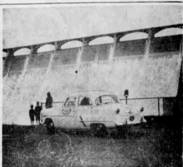
Frothing as it cascades down 500 feet, water from Franklin D. Roosevelt lake pours over spillways at Grand Coulee dam.
