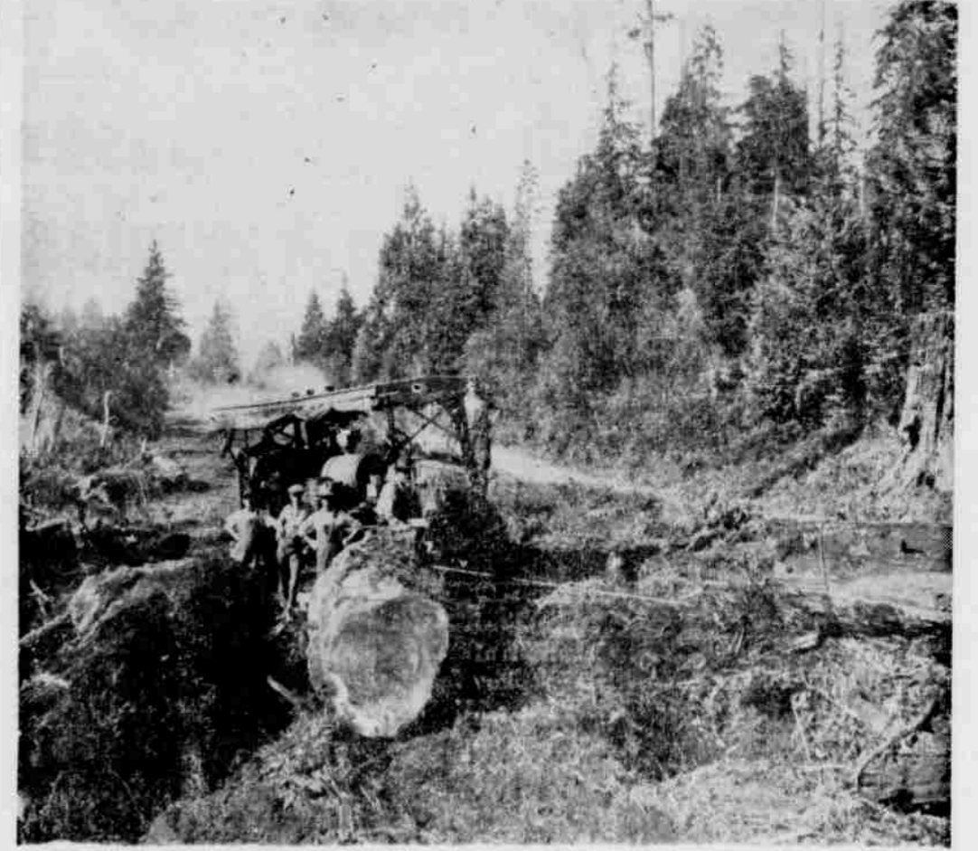
When contractors started building state highways some 33 years ago they moved logs off the right-of-way by just rolling them along the best way they could figure. Now they push them aside with bulldozers like elephants in the circus, quicker and easier. (Oregon State Highway Commission photo).
