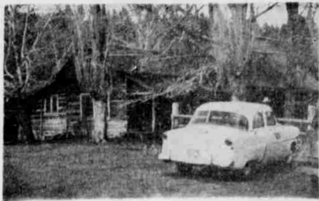
Old Williams ranch house on Canyon creek, with white Oregon State Motor association car parked in sideyard. Timbers for house, built in 1860s, were hand-hewn with dovetailed corners. Mammoth poplars and silver maples were brought in and swelled by pack horse. Today, they serve to shade entire dwelling.
