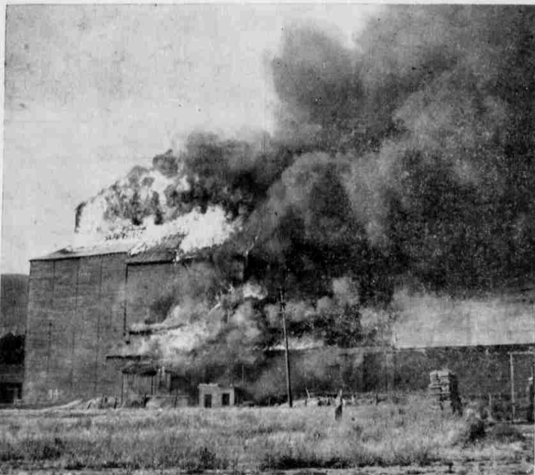
NOT ONLY FLOOD, BUT FIRE too, has played its part in Heppner's history. This spectacular blaze was one of the most recent, and one of the most destructive to hit the town. On the afternoon of July 18, 1949 the elevators of the Morrow County Grain Growers, and one owned by Interior Warehouse, located on the railroad in the west end of town caught fire. Shown above is what Heppner firemen, aided by equipment from Lexington, Ione, Arlington, Ordance, McNary and elsewhere had to face on that hot summer day. High winds scattered the flaming embers and for several hours threatened to wipe out a big section of the town before being brought under control. Loss was estimated at over $600,000, but no lives were sacrificed. Much of downtown Heppner was burned in a big fire in 1918, but no pictures of this catastrophe could be located.
