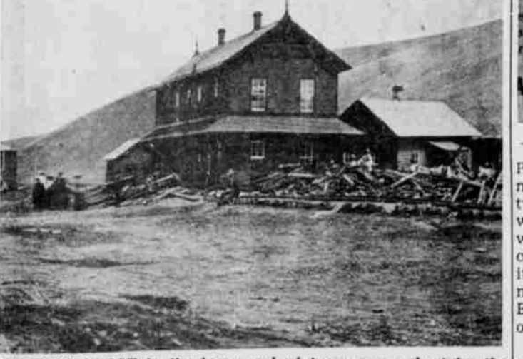
HEPPNER DEPOT in the lower end of town was unhurt by the waters, though it was well surrounded by debris after the flood receded. The building still stands and is still being used for the same purpose, though remodeling has changed its appearance slightly.
