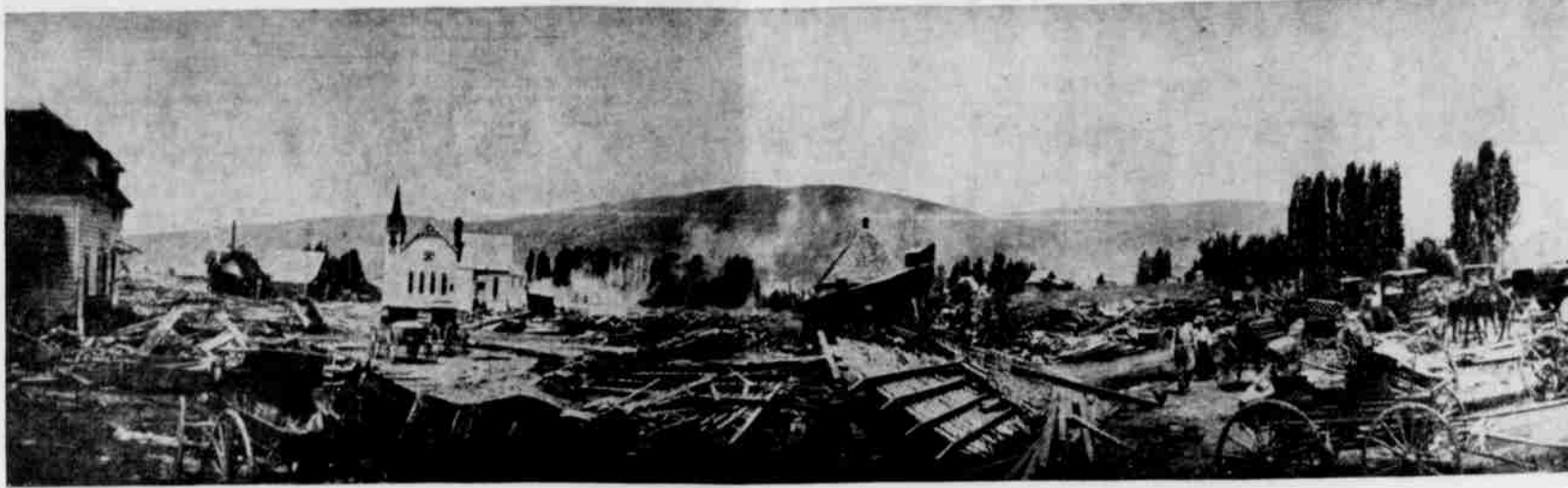
ONE OF THE BEST GENERAL VIEWS of the great destruction caused by the wall of water, is shown in this old photograph. The white building on the left with the steeple is the Methodist church which still stands in the same location. To its left, in front of the barn and leaning against the angled telephone pole that
