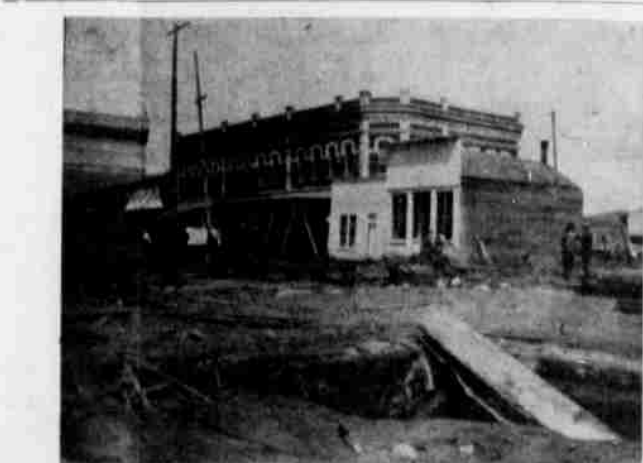
CASE APARTMENT BUILDING is in the background in this picture taken from approximately where the Morrow county creamery now stands. Nearly everything between this building and the creek, about two blocks, was washed away.
