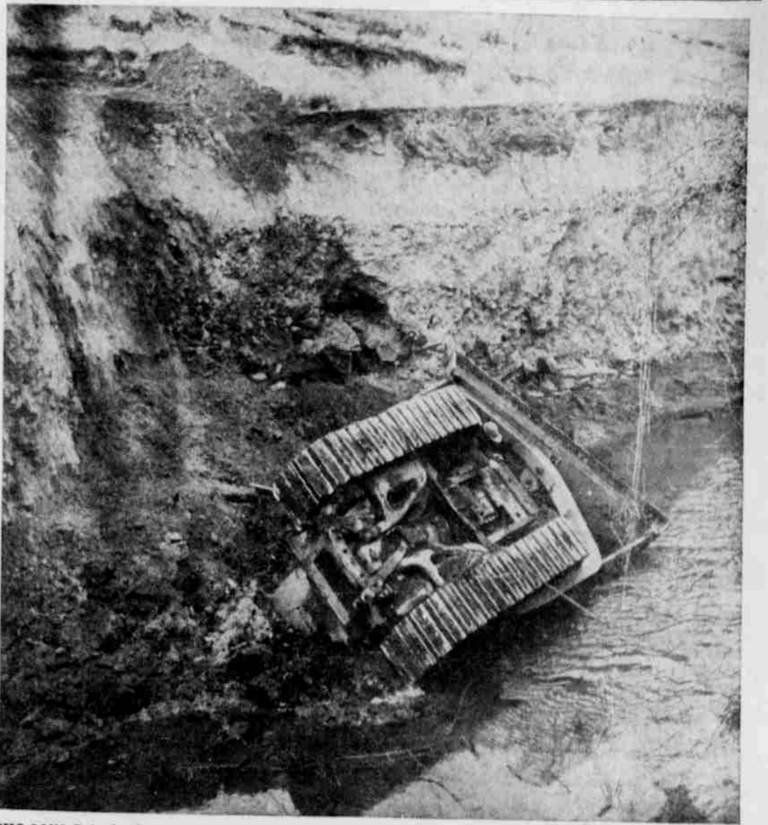
WHO SAYS Cats don't take to water! This Cat (erpillar) driven by Terrel Benge went for a swim in Rhea creek last week when a section of bank gave way under it. Benge, who was unhurt, felt the ground slip and climbed off to watch it slide down the bank and tip over, winding up in the position shown in the picture taken by C. A. Ruggles. Neighbors aided in righting the tractor which suffered only minor damage from the spill.
