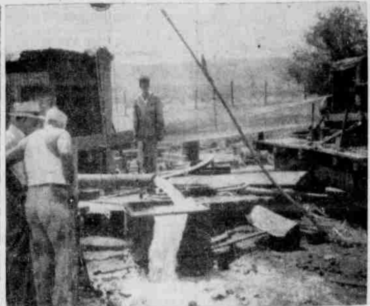
WATER —Worries disappeared in a hurry Tuesday when water began pouring from the pipe of the new city well. Present to watch the test made by employees of A. A. Durand, Walla Walla well driller were most of the members of the council and several other interested citizens. The well was given a five hour test and produced a sustained flow of 361 gallons per minute, sufficient to supply practically all the city's needs. Temperature of the water at the pump is 54 degrees, which gives promise of considerably cooler water from the tap. (GT Photo)
