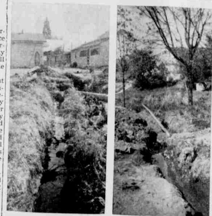
TO BE ELIMINATED—These open sewage ditches are just two of the many that will be eliminated with the completion of the sewer system Heppner voters approved Tuesday. These pictures were taken over a year ago when the project was still only in the discussion stage.
