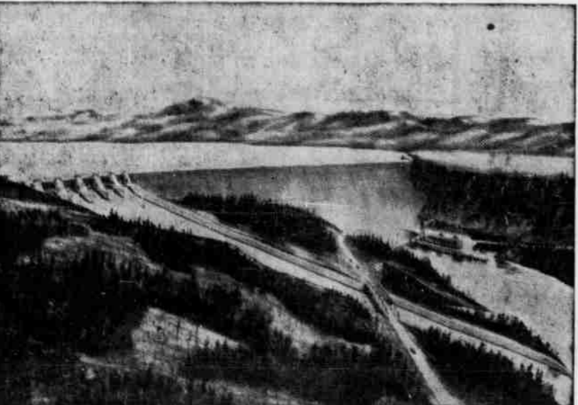
ARTIST'S SKETCH shows how Yale will look on completion. Spillway section at left will be concrete, main section will be rock fill. Generators will be in powerhouse at right. Yale Project, operated in tandem with Merwin plant downstream, will produce an estimated 550,000,000 kwh. of electricity annually.
