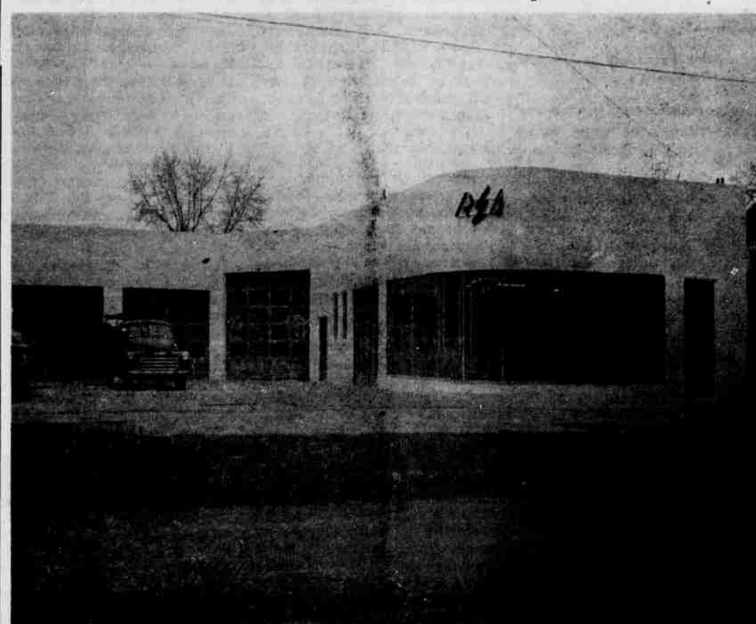
This is a picture of the REA building before the windstorm Wednesday night. The seven big panes along the side and front of the office were reduced to only three good ones after the storm got in its work. The building is so located that the full force of a south wind smacks it right on the glass front. No other damage was done to the building, inside or out.
