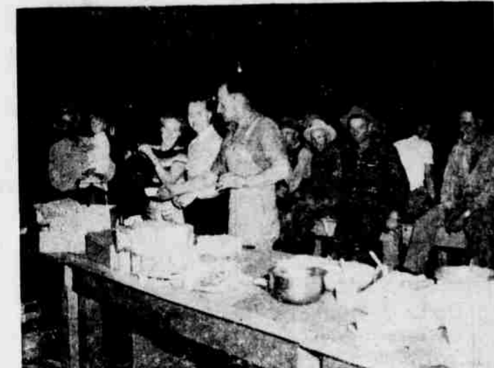
On the Chow Line About the most important branch of the floor-laying party was the chow line, which proves that the men can't get along without the women, even if they
