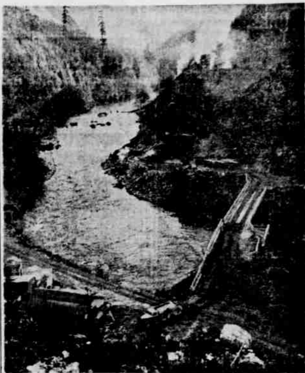
Looking down from new highway on dam site near Detroit.
