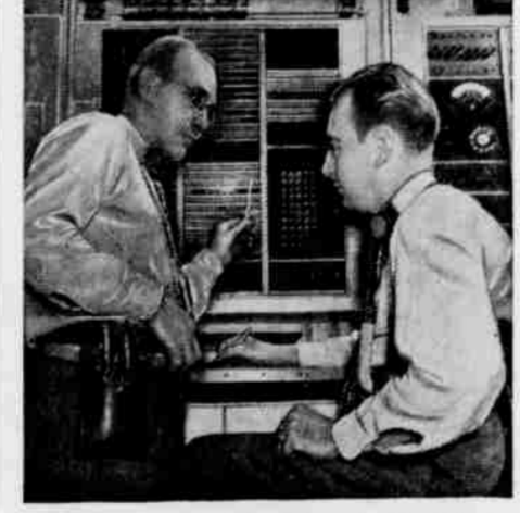
3. On-the-job-training here in the West is typified by this "student" who is learning the workings of a trouble indicator frame—an automatic detective that constantly makes sure the lines on its "beat" are giving good service. Even experienced employees take refresher courses like this to keep up-to-date... and keep learning their way up the ladder.
