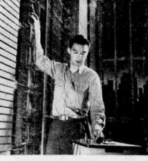
2. One important night-time job is done by this electronic tester. It checks lines to make sure they're in good shape. At the same time, other telephone men are vacuum cleaning and inspecting sensitive switching equipment . . . you might say it's stopping trouble before it starts. And night is the best time to do it, while most telephone users are sleeping. 4. The real value of telephone
