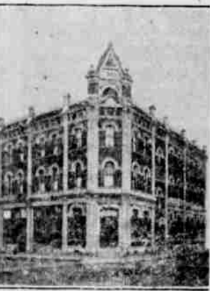
Some of our readers will see nothing familiar about this picture, but to older residents it will be no strange sight. The Palace hotel, built in the early '90's, occupied the corner where the Rosewall garage now stands. It was the meeting place of ranchers, traveling salesmen, business men and—just folks. Fire broke out in the hotel on July 4, 1918, destroying the building and contents and before being brought under control spread to the blocks to the south and burned out most of four blocks.
