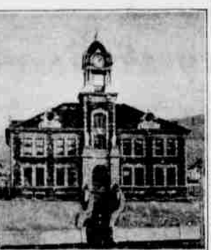
Built of native basalt rock and trimmed with Wallowa county sandstone, the Morrow county courthouse has long been considered one of the better buildings of that type in this part of the country.
