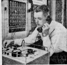
1. Your voice gets a boost in repeater sta tions like this one. For currents fade on the lines and without amplifiers, your voice would soon be lost. The equipment can literally turn faded voice into a roar. Much of it requires only periodic check-ups like the one the technician is giving it here.
