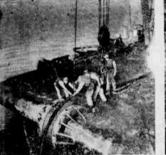
2. On the job fast, a repair barge grat for the cable and lifts it from its under bed ... guided almost to the exact spot by me distant test center. And the moment the break was discovered, other telephone people in the Traffic Control Bureau set up emergency routes to make any delay on your calls as brief as possible.
