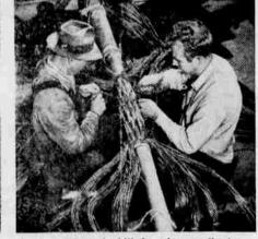
3. At top speed, skilled workmen splice in a new section and the cable is soon back in service. Although there are hundreds of underwater crossings in the West's many bays and rivers, such emergencies are infrequent. But telephone people are on the job 24 hours a day to keep your telephone ready to work for you any time you need it.
