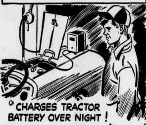
WITH NEW SELENIUM-RECTIFIER-TYPE OVERNITE CHARGER DEVELOPED BY GENERAL ELECTRIC BATTERY IS CHARGED WITHOUT BEING REMOVED FROM CAR OR TRACTOR.
