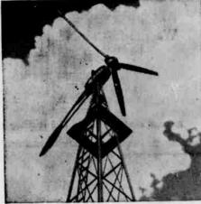
Above the desert floor we sometimes wind-driven generators to supply power for long distance amplifying stations miles away from electric lines. When the wind dies, gasoline motors take over to charge the batteries at these repeater stations that give a "boost" to your voice as it journeys with the speed of light
