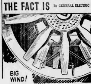
600-M.R.H. HURRICANE IS CREATED IN THIS WIND TUNNEL AT MOFFETT FIELD, CAL. IT TAKES GENERAL ELECTRIC MOTORS TOTALLING 27,000 HORSEPOWER TO TURN THE BLADES SHOWN IN THIS PICTURE.
