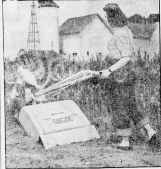
The new Rototiller farm machine, produced by Graham-Paige Motors in the giant Willow Run plant, prepares soil for planting in a single operation, making unnecessary the three operations of plow, disk and harrow. The five-horsepower tiliage unit, which churns and crumbles the soil to a depth of nine inches, has attachments which adapt it to a score of other farm tasks such as huildozing, seeding, mowing, snowpiowing and other operations.
