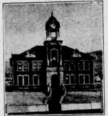
The modern court house of today, a stone structure built in 1902. Some native rock was used in the structure.
