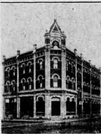
Heppner's once famous hostelry, razed by fire in 1918. Phil Metschan and J. L. Wilkins were noted hosts. It stood on the site of the first trading post, conducted by Henry Heppner and Jack Morrow. This site on the northeast corner of Main and May streets is now vacant.
