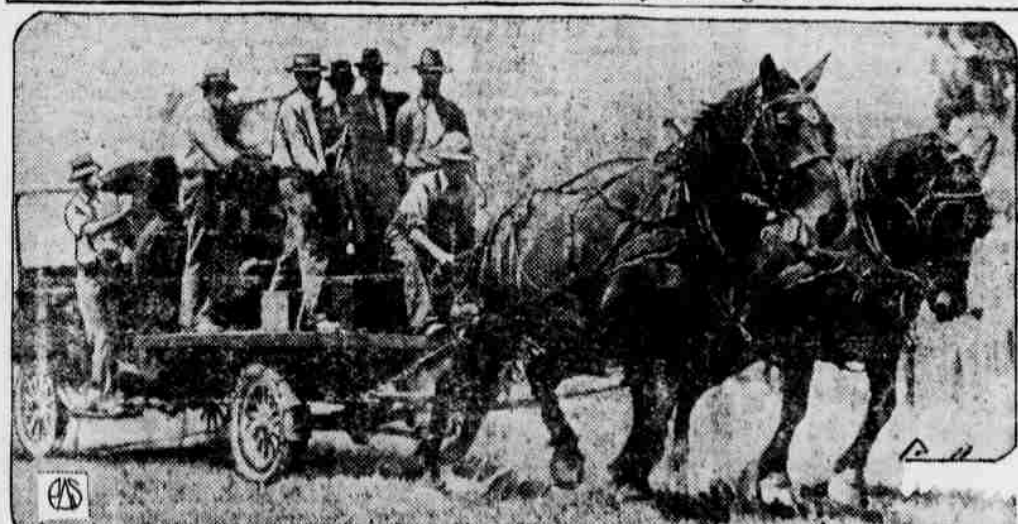
"Bill" and "Colonel," the 3,800-pound team belonging to George Wilcox, of Greenville, Ohio, pulling against a motor truck, at the Jay County, Indiana, fair, made a record of 3,550 pound drawbar pull, equal to hauling 40,102 pounds on a wagon or eight fourteen-inch bottoms cutting a furrow six inches deep.
