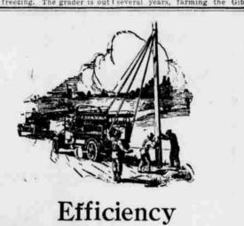
OWN the road it travels, one of the most efficient things on wheels. Coils of wire are stored inside. Tools are in the snug lockers. Pike poles and shovels are in their racks. A big winch is bolted to its frame and there are pipes of steel from which to form a sturdy derrick.
