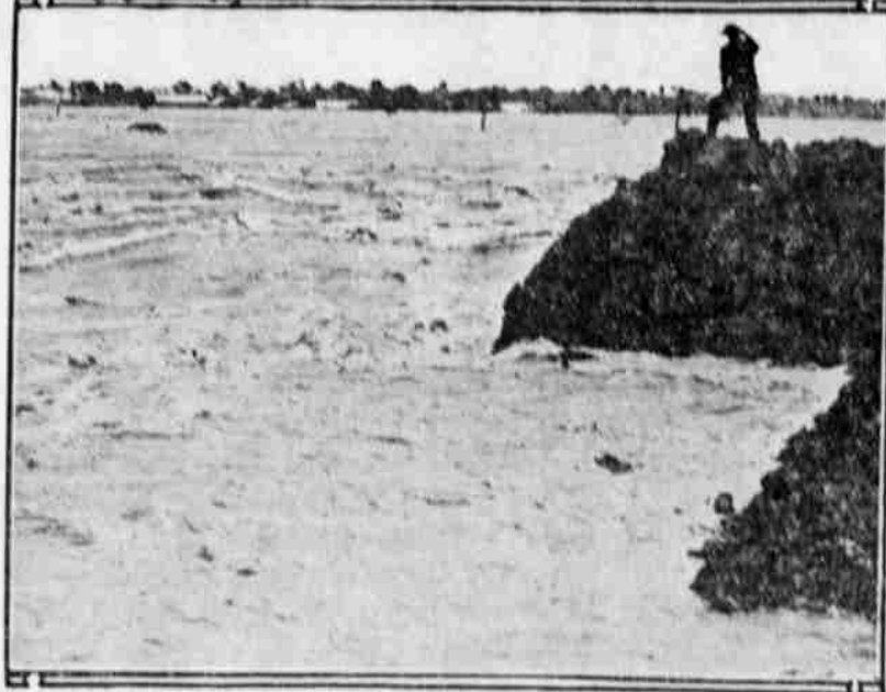
Flood Waters Raging Through a Break in a Mississippi Levee.
