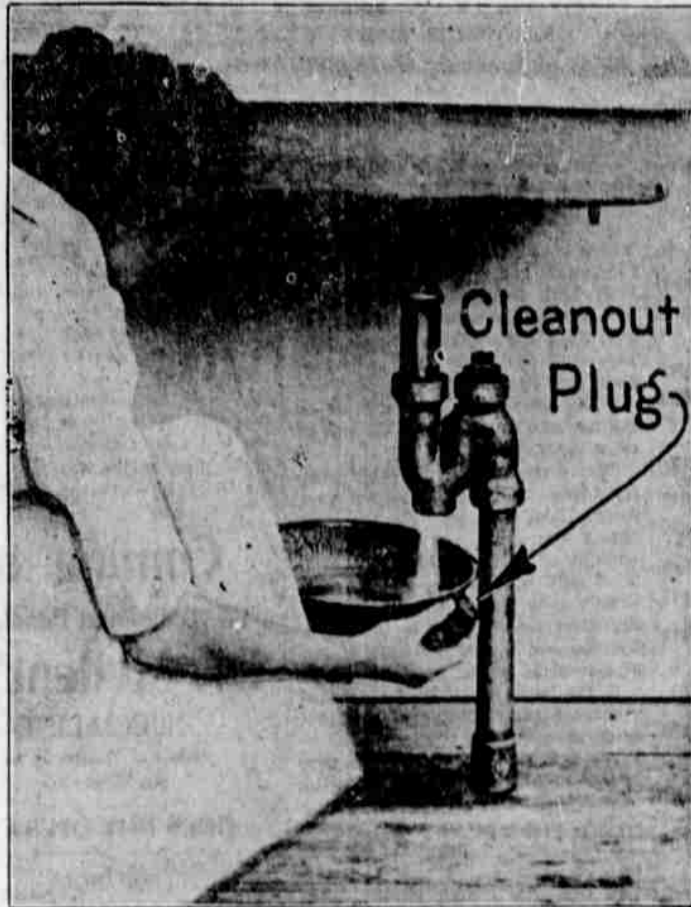
Cleaning Out a Sink Trap.
