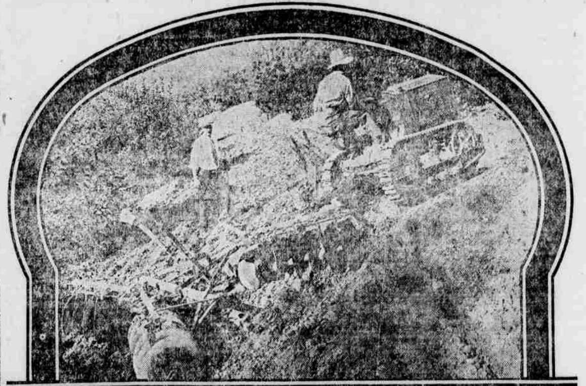
Cleveland Tractor with tandem disks working on 20% grade.
