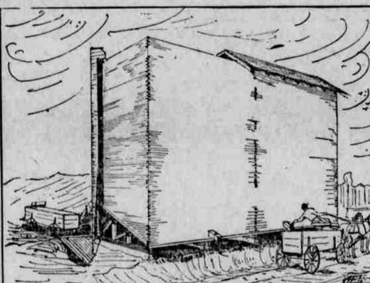
Design X-103—5000-bu. Stationary Grain Bin. All lumber necessary to build, for \$282.00.
