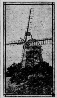
tion of the milistones the whole structure, including the machinery, is of wood. All the cog wheels are cut from native hard maple.
