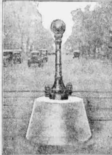
This Street Signal Has the Usual Large Red Globe and Two Additional Smaller Red Lights Near the Base, to Indicate a Railway Crossing.
