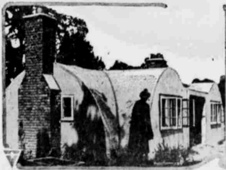
An experiment is being made in Buckinghamshire, England, of building attractive houses with concrete. Constructed as bungalows, the interiors present a cozy appearance with vaulted roofs which will make them delightfully cool in the summer and warm in winter. Absolutely water-proof houses can be constructed within two weeks.
