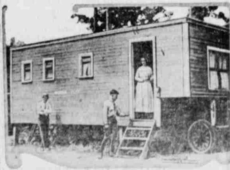
William Travers of Jacksonville, Fla., returned from war only to find that he could not obtain a home for himself and wife. Being an engineer and contractor, he bought a used army auto truck, obtained some lumber and built a three-room house on it. Now Mr. Travers and his wife can live wherever they wish, and are free of paying landlords. The house is provided with gas, electricity and water fittings for connections.
