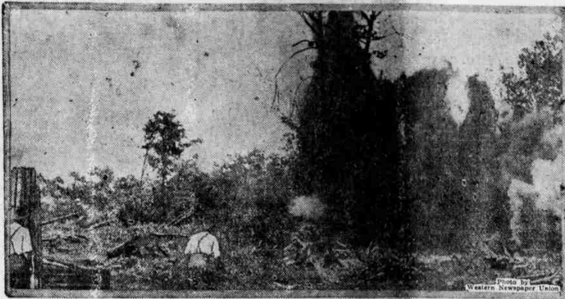
At Newark, N. J., a small army of men is busily engaged in clearing Heller field which, when completed, will be the first United States aerial mail landing field in the country. Our photograph shows the moment of detonation of a charge of dynamite beneath a mighty tree stump, which is torn from the grounds, roots and all.
