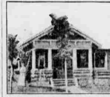
In This Pretty Bungalow the "Logs" Are Precast Concrete Units, Laid Up With Mortar, Like Any Masonry, and Stained Wood-Brown on the Outside to Look Natural.
