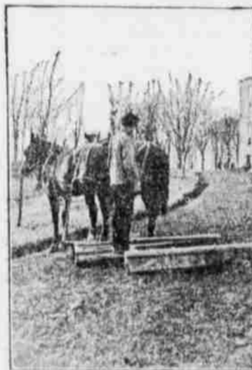
Standing on Drag While in Operation. amount of cutting done by the front runner and when to lengthen it in order to produce the opposite effect.
