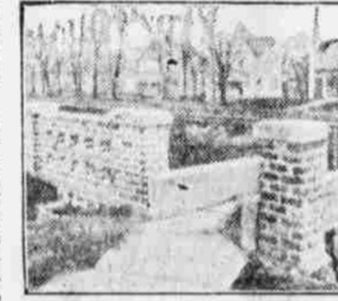
Ornamental Brick Wall Marking the End of a Blind Street in Cincinnati. It Was Built at Small Cost by the City's Engineering Department With Samples of Brick and Cement Submitted for Test Purposes.
