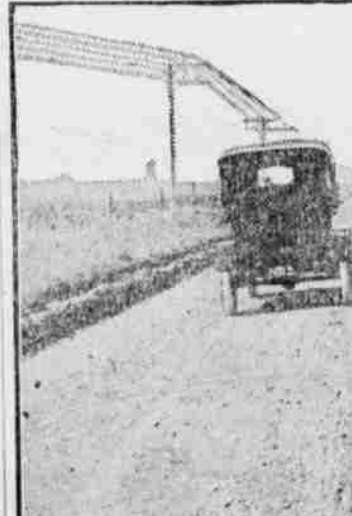
Well Drained Road.
