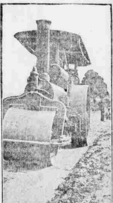
Road Roller Doing Repair Work.
