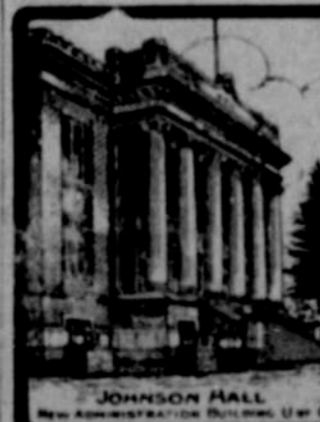
JOHNSON HALL NEW ADMINISTRATIVE BUILDING, U. OF O.
