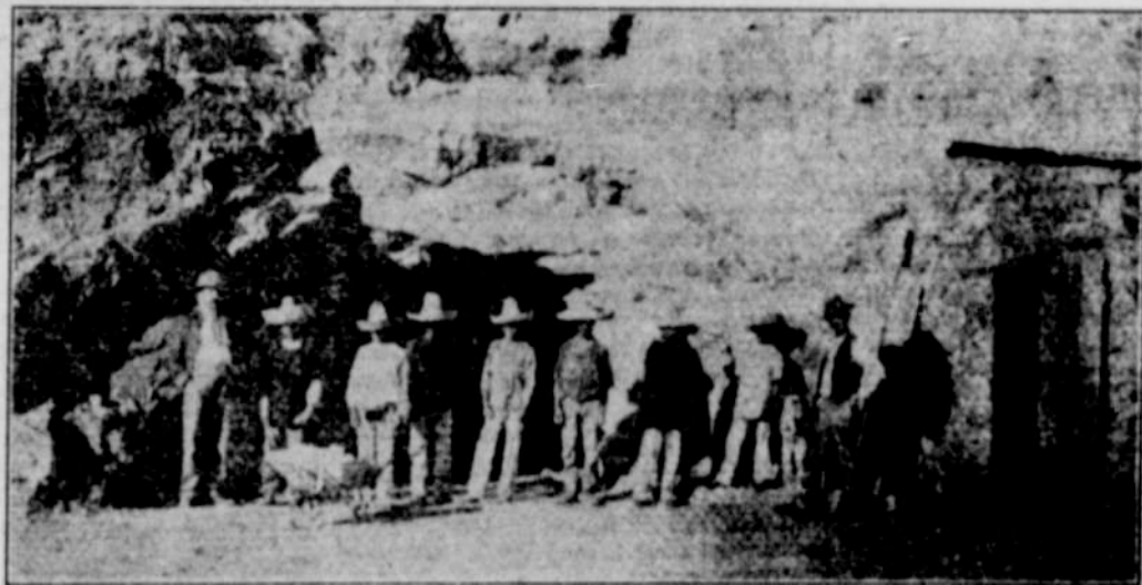
VIEW OF THE MEXICAN MINE LIMITED. WM. EHLERT, MANAGING DIRECTOR, AT THE LEFT AND CHAS. CUMMINS, RESIDENT MANAGER AT THE RIGHT
